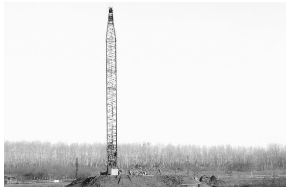
Figure 2. Test site and used crawler crane in the field investigation.
